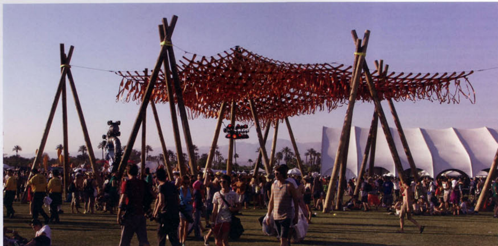
3. Copper Droopscape was a study in non-standard modularity. While it employed a uniform cell dimension, each of its 864 parts was unique. The standard cell made field assembly manageable, while each part's non-uniform aspects – the form and proportions of the hanging tendril – yielded a rich visual and aural experience.
