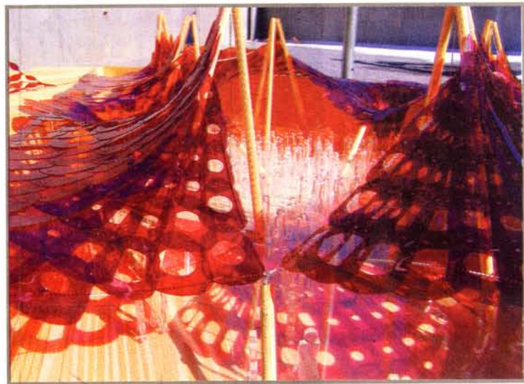
© 2007 The Museum of Modern Art WINNING WAYS: A mock-up of "Liquid Sky," a pavilion slated for the courtyard at P.S.1 in Queens, N.Y., reveals the team's use of Mylar and phone poles to create a vibrant, light-filled space.
