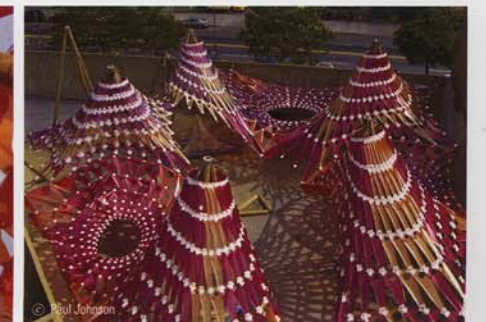
Six towers constructed from utility poles support the surface
